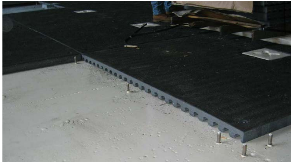
The "M" pattern on the bottom of each panel channels the water aft.
