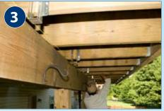
Use a taught stringline between the two outermost rows of brackets as a guide to complete the bracket installation every 24" or 32" (Do not exceed 32" spacing).
