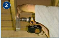
Move to the opposite or drainage end of your deck. Determine proper slope for the panels (minimum 1/4" per 4' of panel length) and install DuoDeck Brackets on outermost joists at appropriate height. (Example: for a 12' panel length—drainage end brackets are installed 3/4" below the "high" end brackets).
