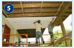
Before installing orient panels label side down (outermost corrugation up). Secure panels with 1" WoodTite™ fasteners every other corrugation where corrugation touches 2x2 purlin. Overlap panels by one corrugation. (26" panels overlap to provide 24" net coverage per panel.)
