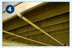
Slide 2x2's through inside of each row of brackets. Secure with two 1" WoodTite™ fasteners per bracket. You'll now see even level rows of 2x2s every 32" (or 24") which gradually step down in height for desired drainage slope.
