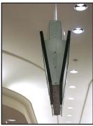
The damshell design presents two halves, one slightly smaller than the other. The sides slip into one another and are secured by a thin extrusion. Depending on the location within the store, signs can be single- or double-faced.
