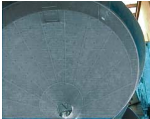
Polystone® Matrox™ liner installed in conical hopper
