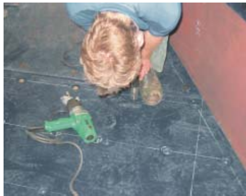
Using a stud welder to attach liner
