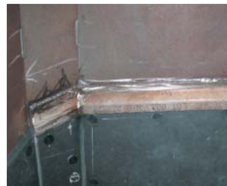
A metal edge protector prevents the bulk material from getting behind the liner
