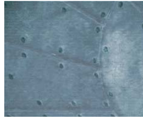
Liner seams are welded
