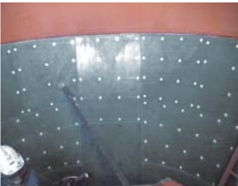
Hopper liner installation
