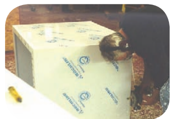
Seams are routed to leave a smooth, clean joint
