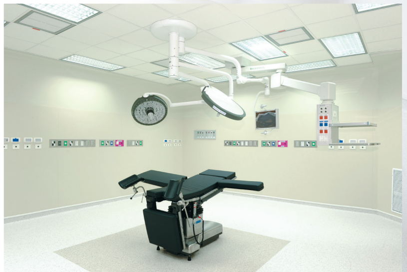
Project: Operating Room
